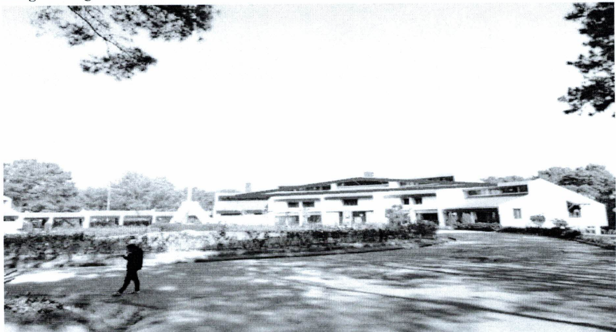
Image 2. A gable-form was hidden in the main building
